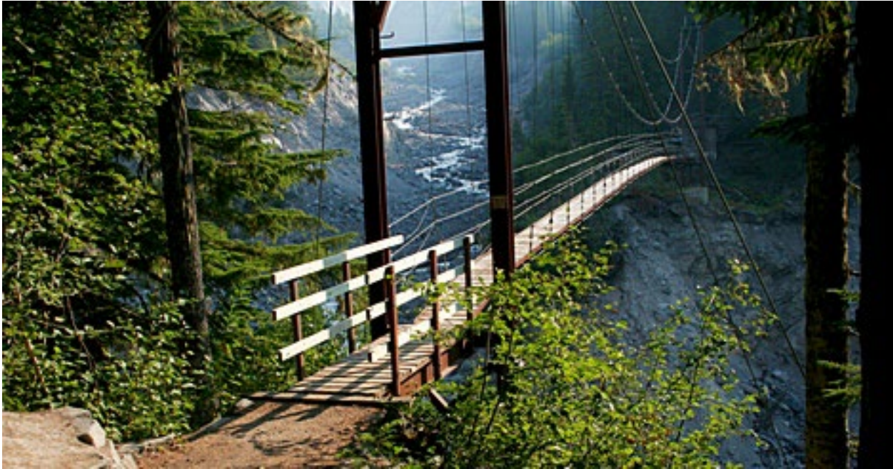
Suspension bridge in Mount Rainier
